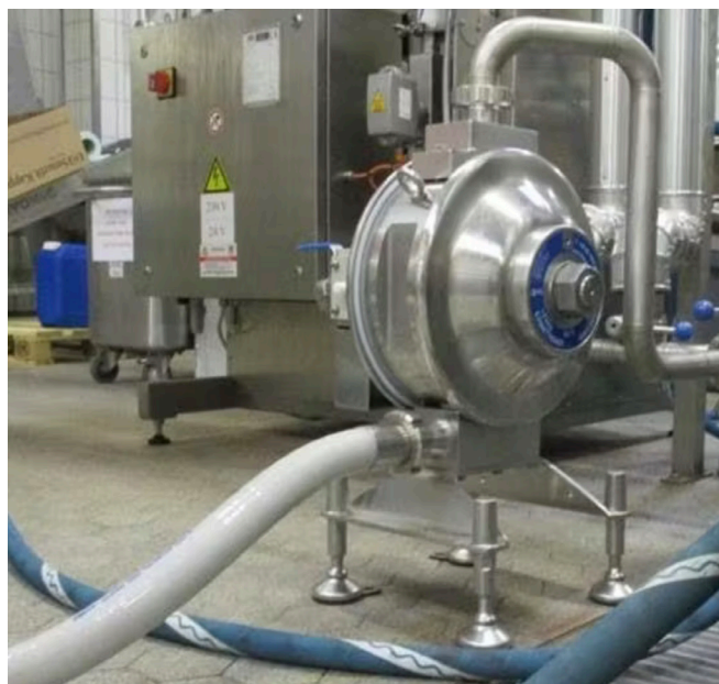
Figure 2: The Flotronic One-Nut AODD pump from Unibloc Hygienic Technologies is an example of a pump design that offers lower internal friction by eliminating pump external pipework.
